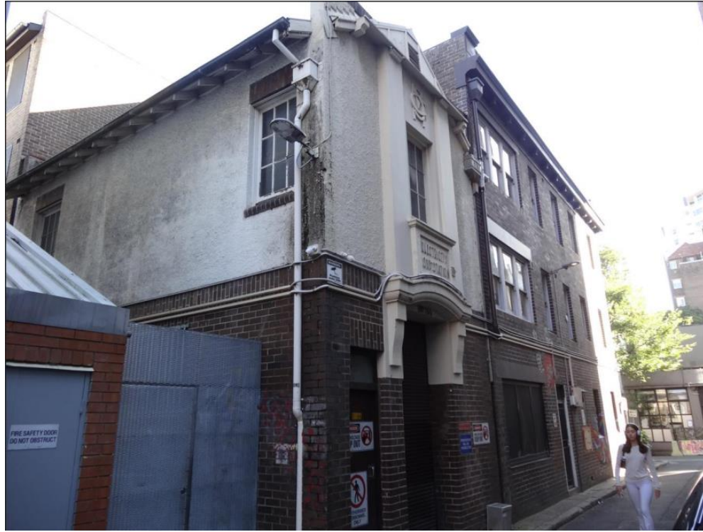
Figure 24: View of the frontage of 1 Orwell Lane (Source: City of Sydney Local Planning Panel Report 19 July 2023)
